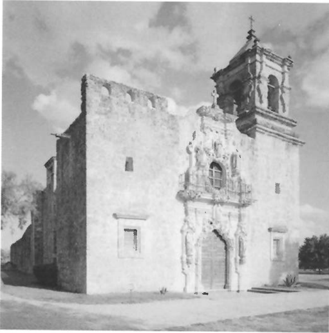
Mission San Jose y San Miguel de Aguayo, San Antonio, TX (1768). Photo: Jet Lowe, HABS, Library of Congress from the forthcoming Buildings of Texas.
