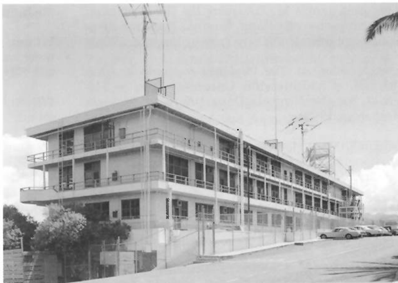
Commander's Headquarters, Pearl Harbor, HI (1941). Photo: Jack Boucher, HABS, Library of Congress from the forthcoming Buildings of Hawaii.
