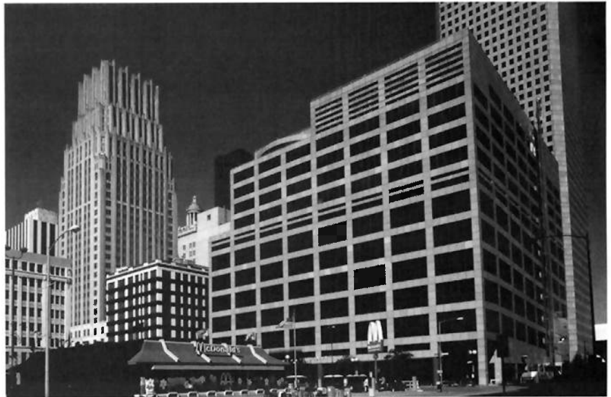
Study in Contrasts: Houston's downtown offered annual meeting attendees a three-dimensional sampler of 20th-century commercial architecture, including the Gulf Building (left, A.C. Finn, K. Franzheim, J.E.R. Carpenter, 1929) and the Texas Commerce Center and Tower (right, I.M. Pei + Partners and 3D/International, 1982 and 1981, respectively), and, of course, McDonald's. Photograph by Christian F. Otto.
