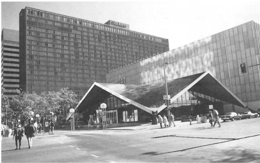
Zeckendorf Plaza, Denver, Colorado. I. M. Pei, 1956-60. Photograph by Alan Gass. The hyperbolic paraboloid has been demolished and the May-D&F department store was stripped and glazed. Both were designed by Pei, as was the Radisson Hotel in the background.
