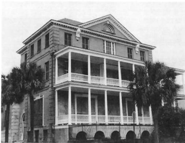
Main facade of Aiken-Rhett House in Charleston showing two-story gallery. Courtesy of Historic Charleston Foundation.
