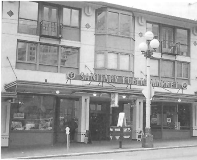
Sanitary Public Market Building of 1909-10. This building was the first in the area to provide extensive refrigeration facilities for the sale of butchered animals, hence its unusual name.
