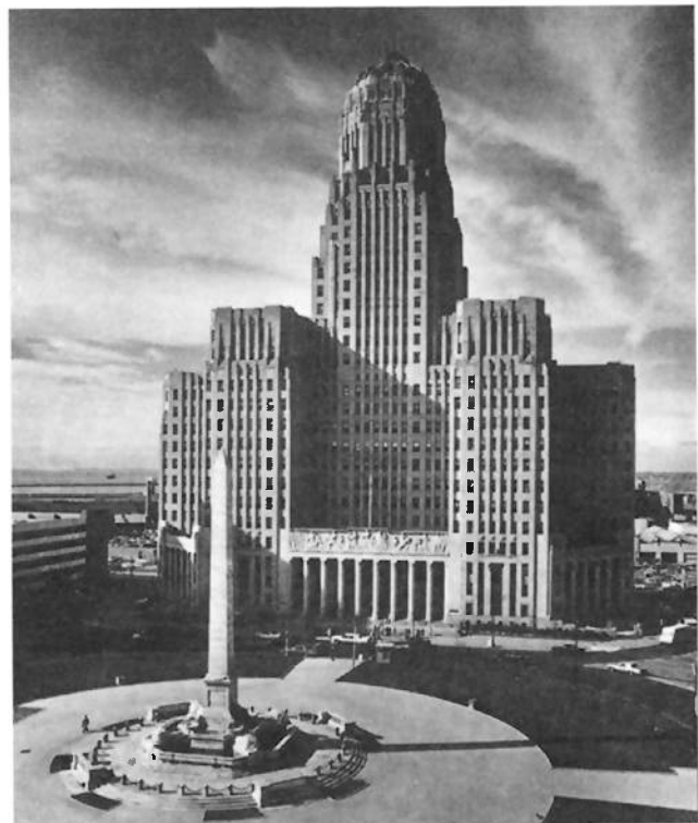
Buffalo City Hall, John Wade, Architect, 1929. Photo by Paul Pasquarello.
