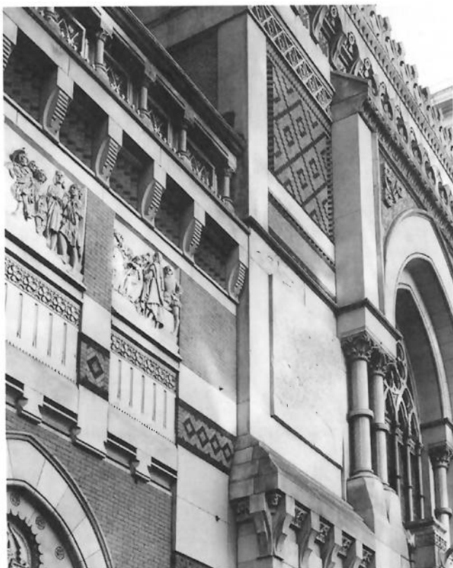
Museum of American Art of the Pennsylvania Academy of the Fine Arts, Philadelphia. Facade detail. Photo by Will Brown.
