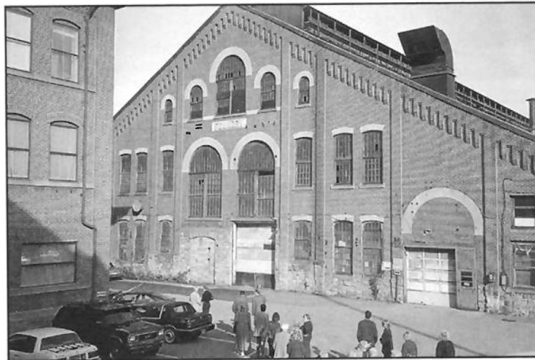
Westinghouse Air-Brake Company airbrake shops (c. 1889), by Frederick Osterling, who also designed important civic and commercial buildings in Pittsburgh.
