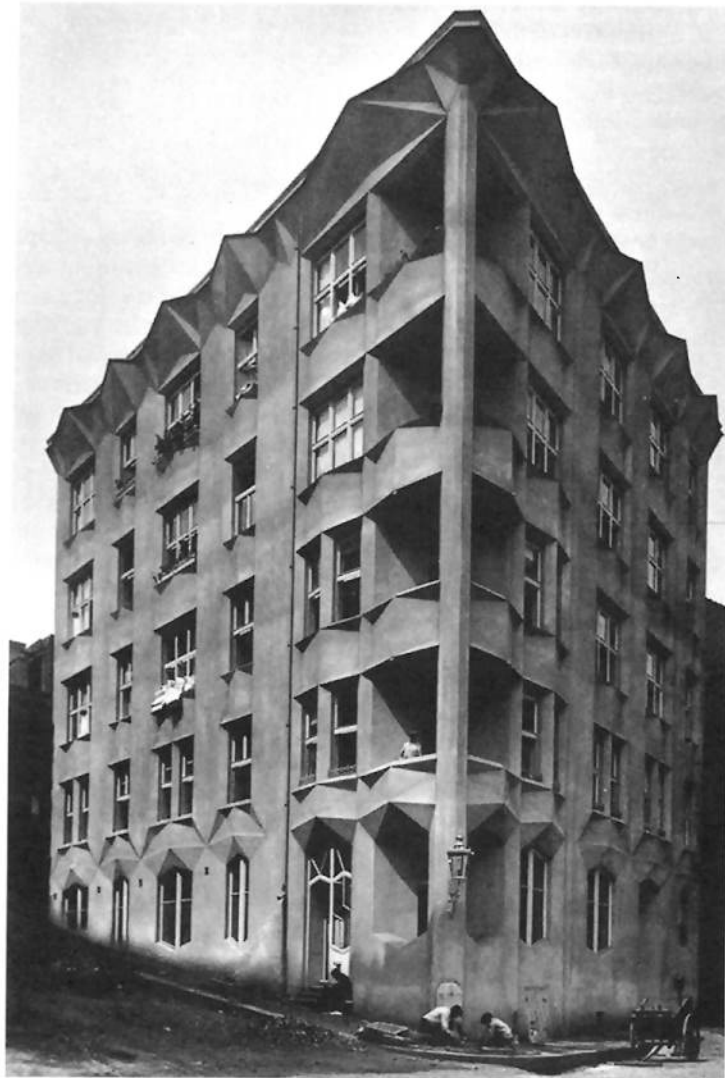
Apartment house on Neklan Street, Prague, 1913. Architect: Josef Chochol. (Collection of the National Technical Museum, Prague)
