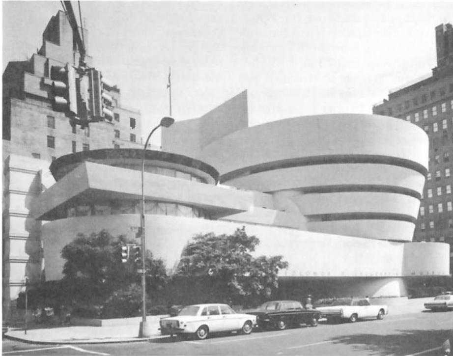
Guggenheim Museum, New York, Frank Lloyd Wright, architect, 1959. (John Bayley, NYC Landmarks Preservation Commission).
